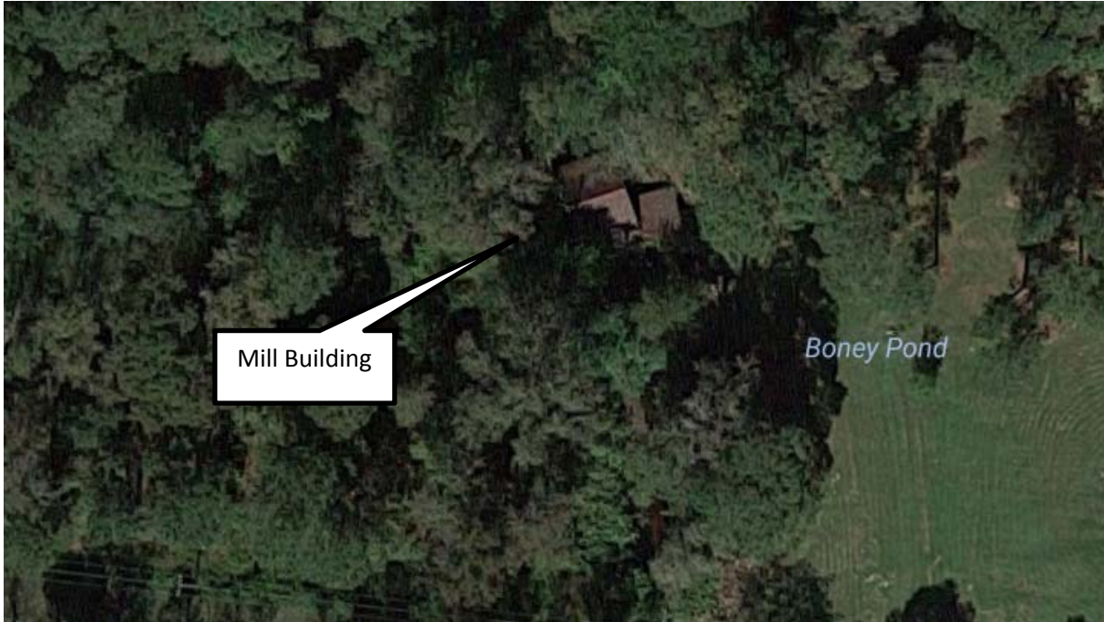
Photo 1: Aerial View of the Vann-Boney Mill (SP0101).
